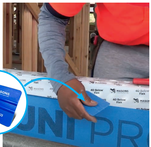
Use scraper for firm adhesion
